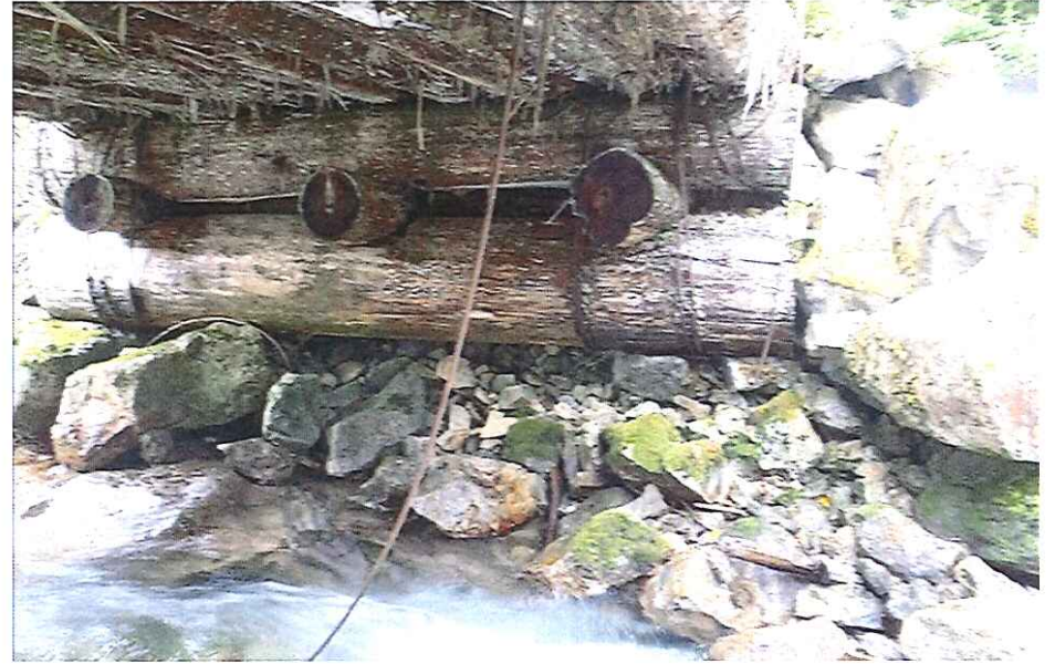
CK 2463 Right Abutment
