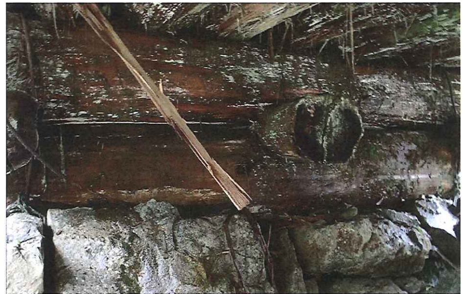
CK2463 Left Abutment
